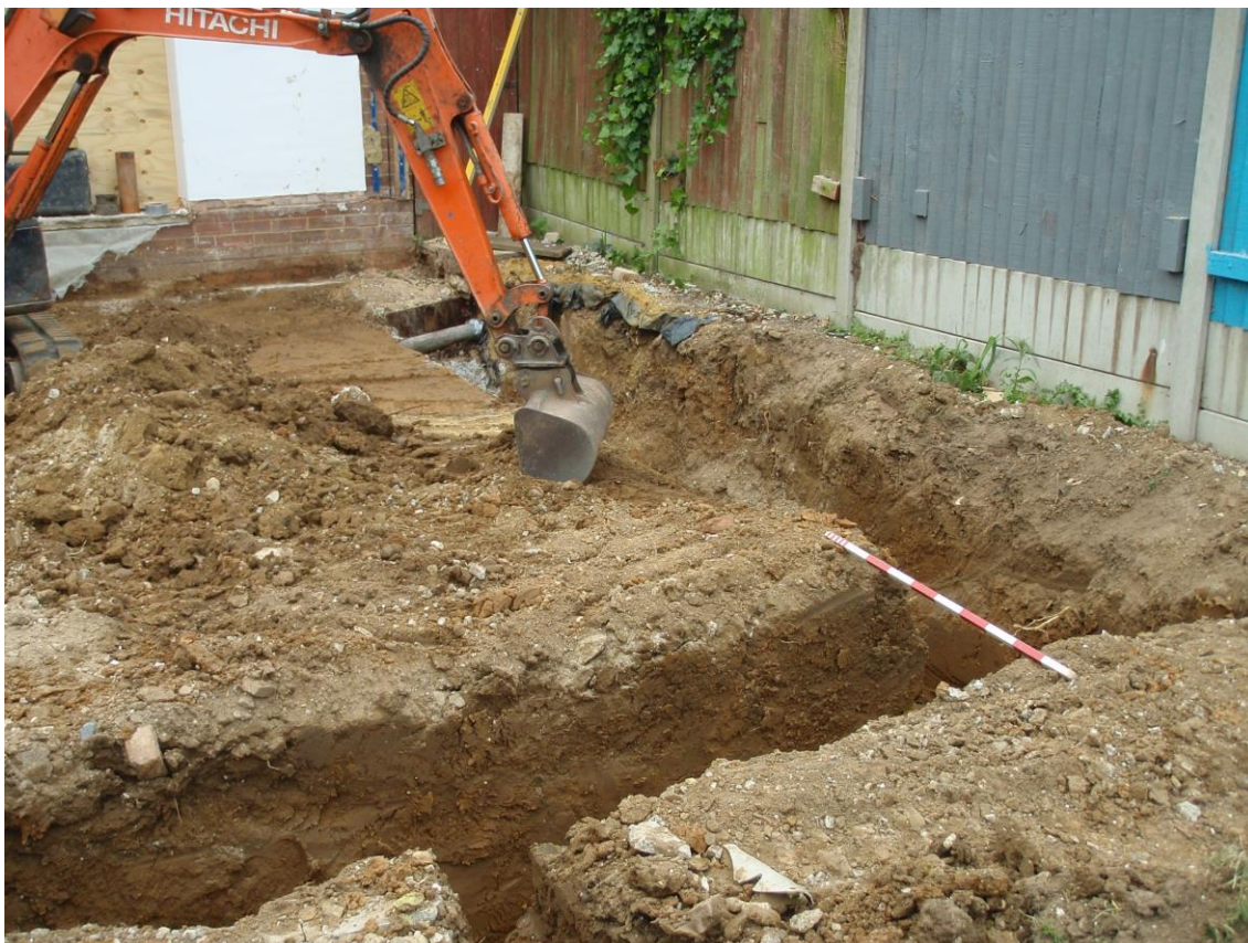
Plate 2. View of trenches (looking NW)
