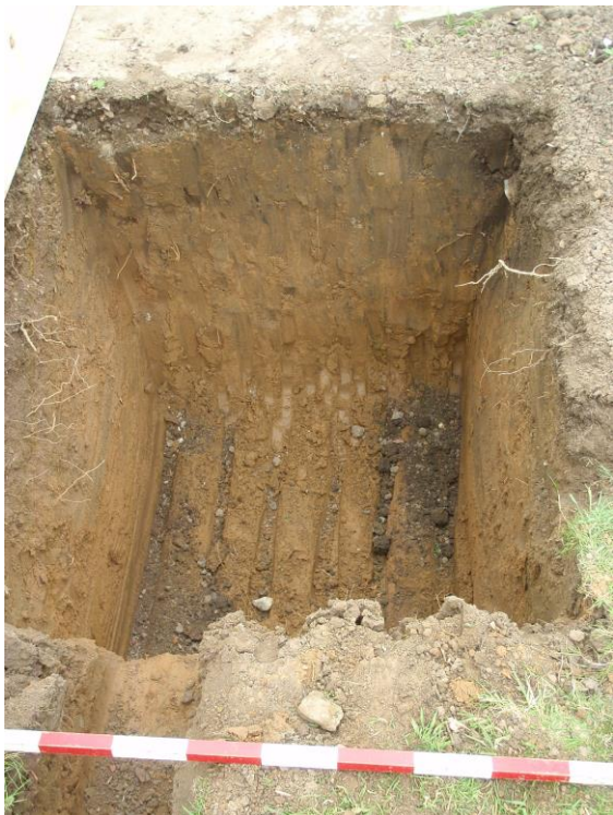
Plate 6. View of soakaway
