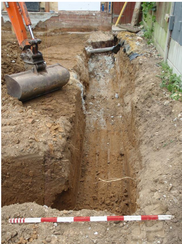
Plate 4. View of north foundation trench
