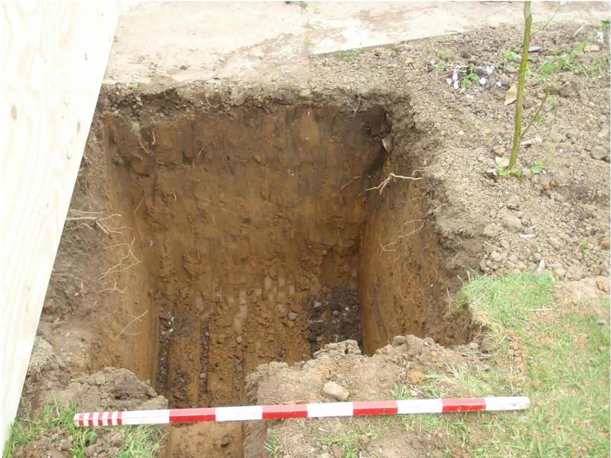
Plate 5. View of soakaway (looking east)
